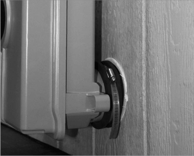
8. Wrap the Metal Bracket Hose Clamp around Flexible Coupling, but do not tighten it.
